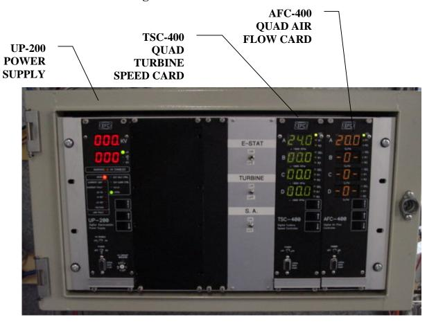
The EFC 4x4 Card cage is a pre-wired system that supports the PS-100, UP-100, UP-200, UP-500, TSC-400, FRC-400, AFC-400 products from EFC. The card cage and back plane can be designed to handle the following configurations:
